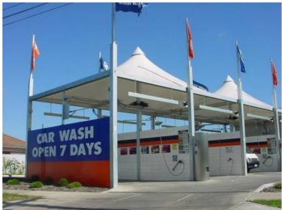
To create a functional and visually appealing structure a double conic roof design was proposed to cover the four washing bays.
