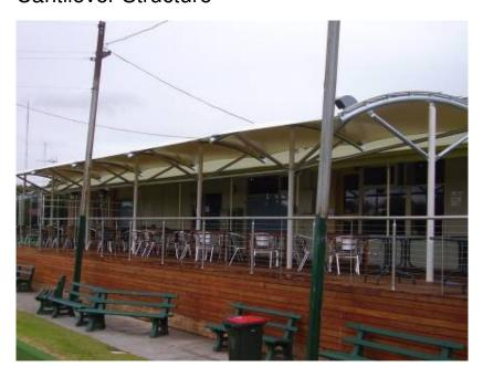
The north facing verandah was renovated to incorporate an extended timber deck and seating area. As part of these works a cantilevered arch structure was installed along the deck area to provide waterproof protection for the new seating area.
