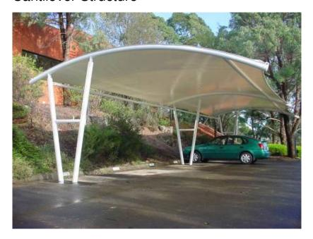
A "V"column cantilevered arch structure was installed at the office car park to protect six car park spaces.
